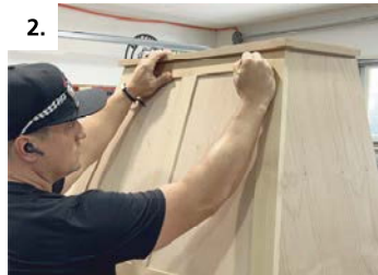
2. Transfer marks from front access panel to upper unit
