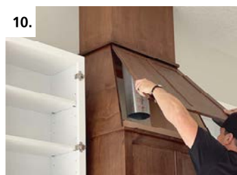
10. Slide top of access panel into place
