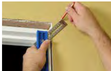
Lay Out Mitered Corners
